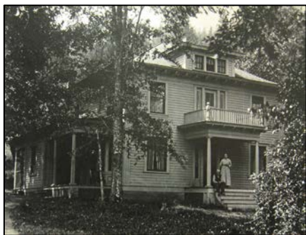
Locke/Galligan House near the time of construction. Photo Credit: Ray Galligan.
